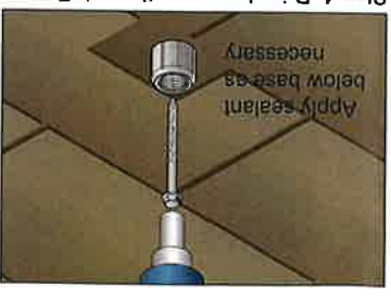
Step 1: Drill rather pilot hole with 3/16" carbide bit
