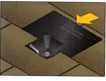
Step 2: Mark trim lines using template and lumber crayon
