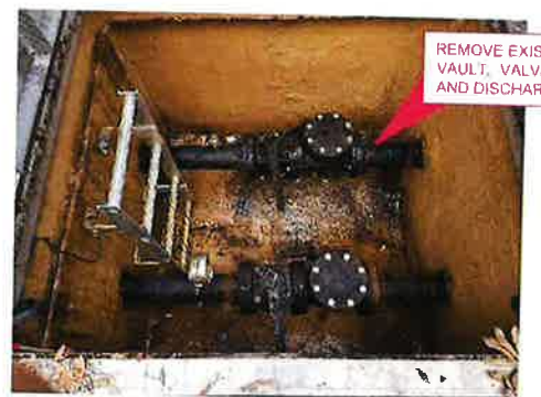
VALVE VAULT AND DISCHARGE PIPING
