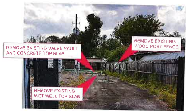
WET WELL, VALVE VAULT, AND FENCING
